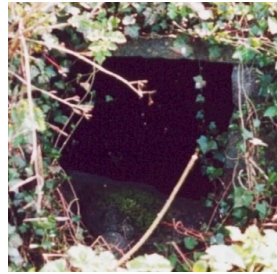
Note stone lined chamber
